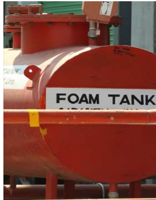
Foam tank for fire suppression
