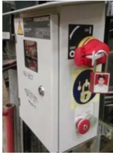
Cut off switch for local isolation
