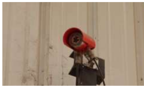
Infrared fire detector
