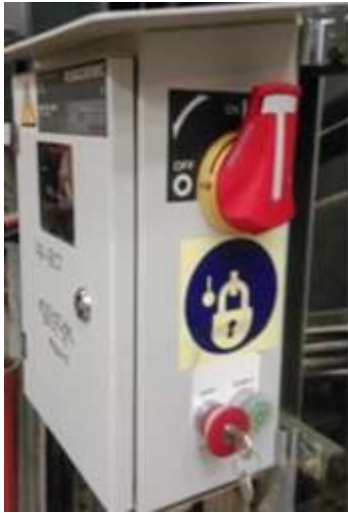
Cut off switch for local isolation
